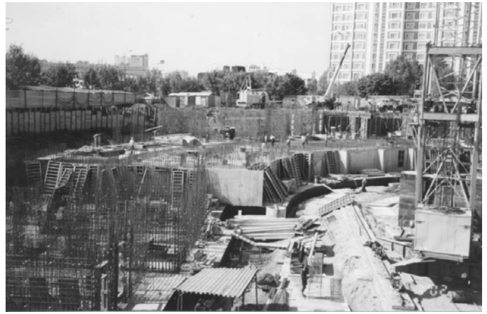
Figure 13. Construction of underground part of the building.
